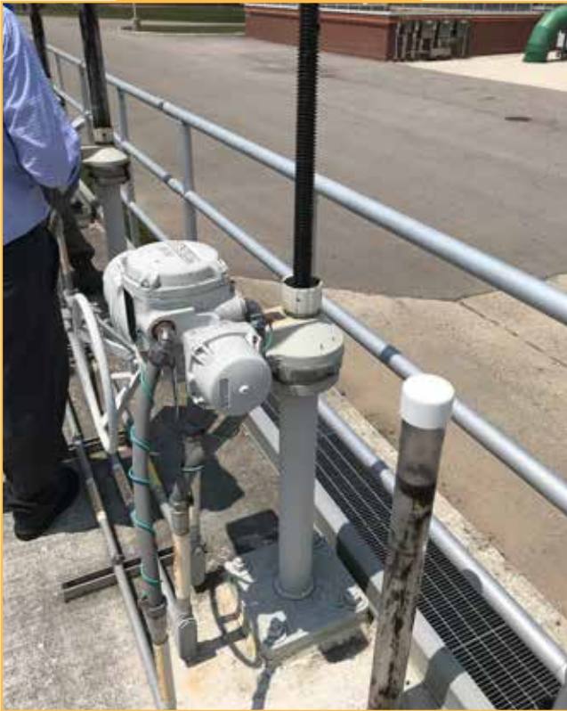
Primary Clarifier Inlet Gate
